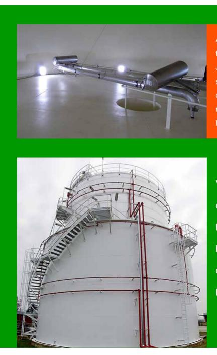
According to IATA standards the tank floating suction ensures the JET-A1 fuel is skimmed from the surface and not from the bottom of the tank thus achieving maximum purity of the fuel being loaded into the aircraft.
